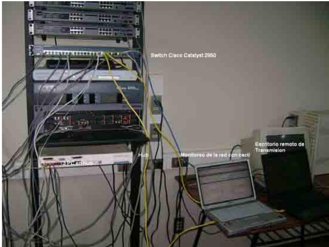
Figura 97. Switch Cisco Catalyst 2950, Hub, Pc de Monitoreo.
