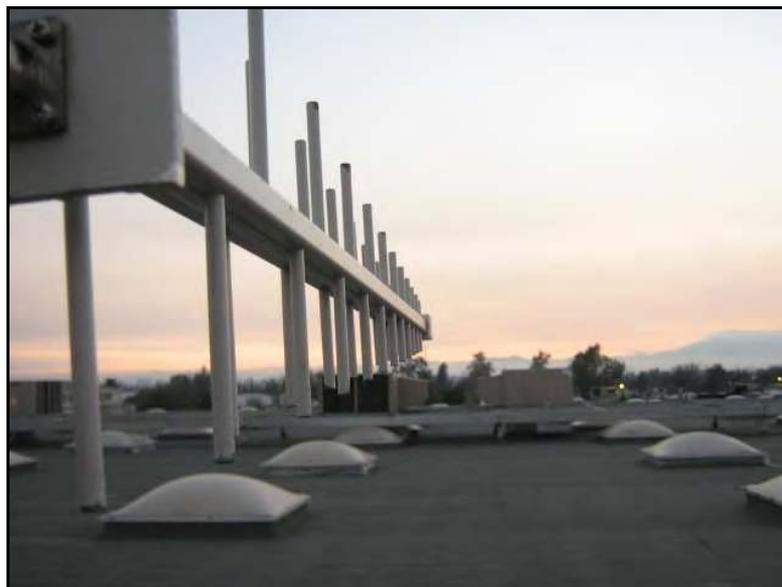
*Figura 35 Antena Yagi Dual band (850-1900).*
