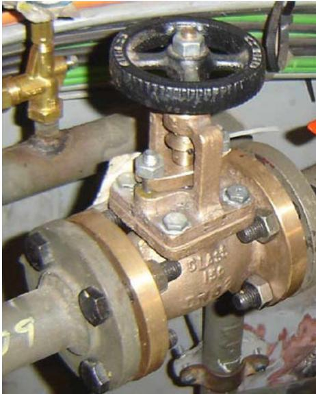
fig 1.10.6 Globe valve with throttle plug
