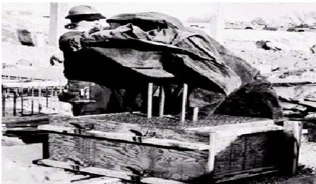
**Fig. 14-8. Concrete footing pedestal being covered with a tarpaulin to retain the heat of hydration. (69870)**
