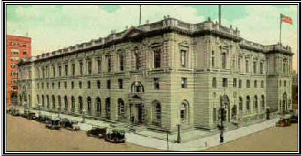
Figura 2.79 Court of Appeals Building, San Francisco (E.E.U.U.).
