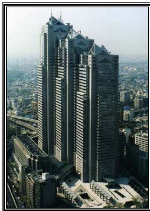
Fig. 4.10 Shinjuku Park Tower.
